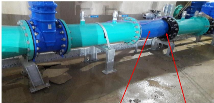
Temporary section of pipe
